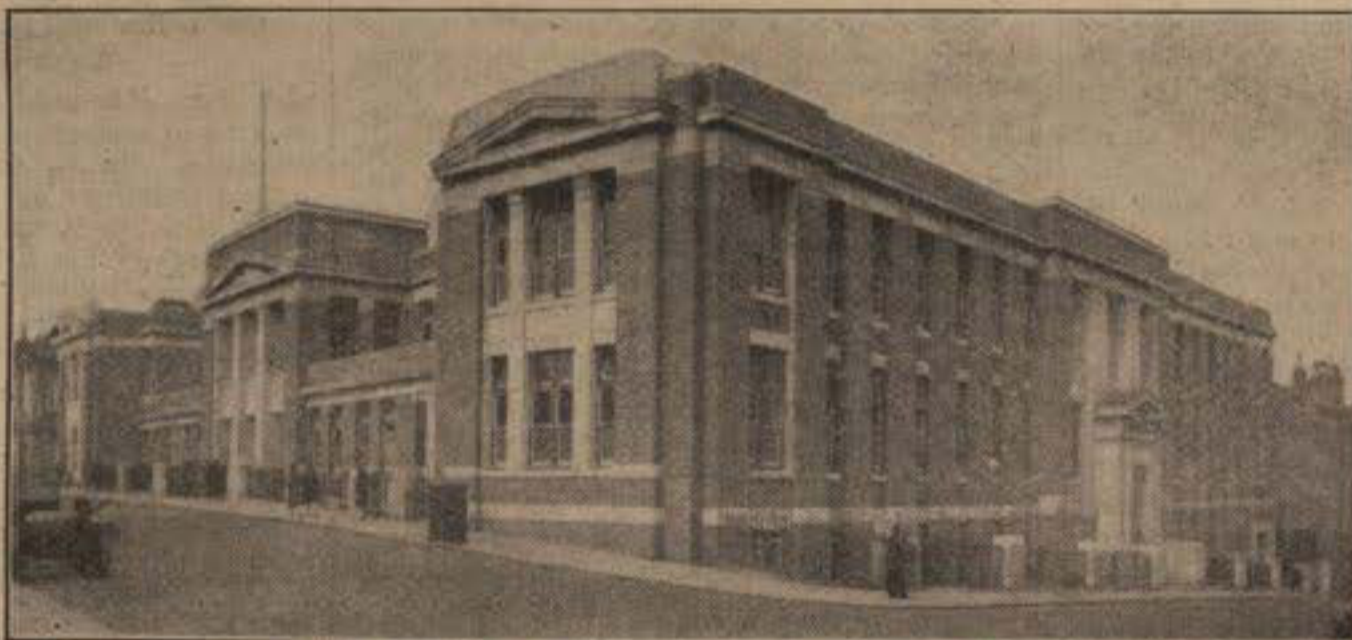
THE NEW WING OF NOTTINGHAM GENERAL HOSPITAL, which was opened by Princess Mary in April, 1927. An appeal on behalf of the hospital will be broadcast from 5GB on Sunday, January 20, at 8.45 p.m.
